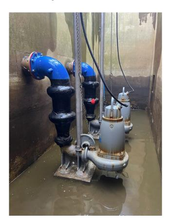
During a routine assessment of the site carried out by the Water Corporation in 2021, it was found that the existing submersible pumps feeding the backwash thickener tank were in poor condition and required replacement.
